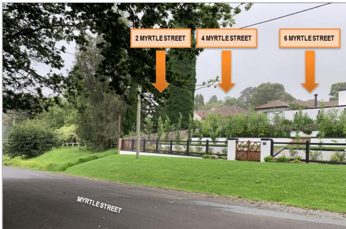
Figure 4: Photo of 2, 4 and 6 Myrtle Street from Myrtle Street (January 2022)
