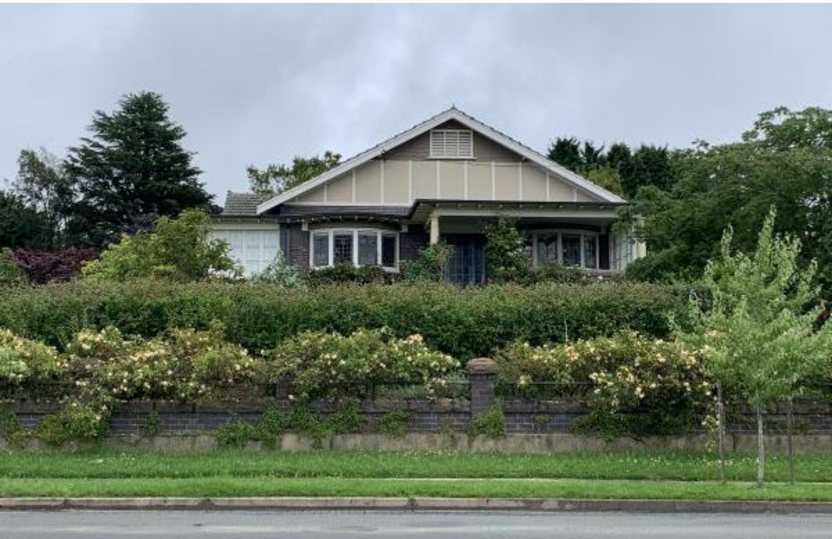
Figure 6: Photo of 'Karingal' from the street showing the gardens and brick & trachyte fence (January 2022)
