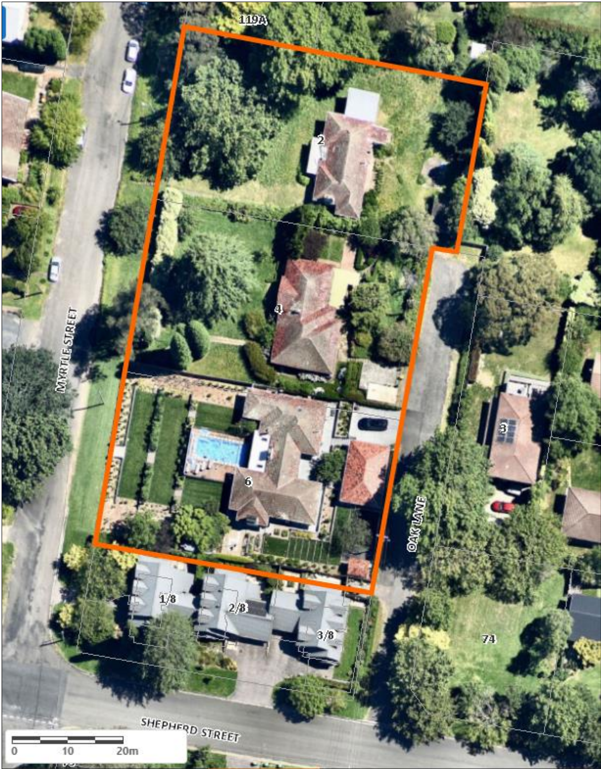
Figure 3: Aerial photo of 2, 4 and 6 Myrtle Street (Source: Nearmap, December 2021)
